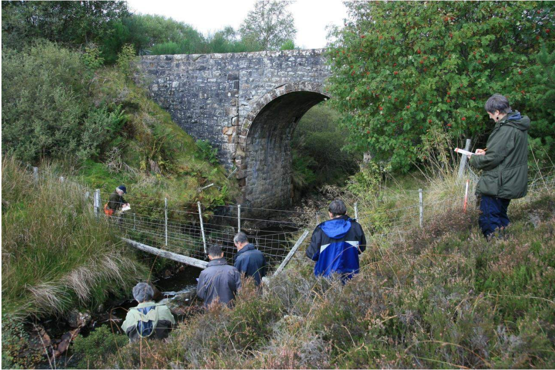
Studying the east face of the Allt na Fearna Mor bridge
