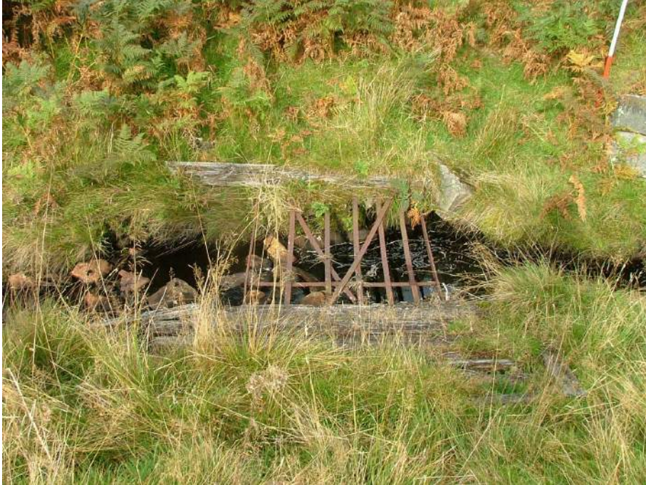
Gate and sleeper bridge at NC 58196 01979 (Mary Stobo)
