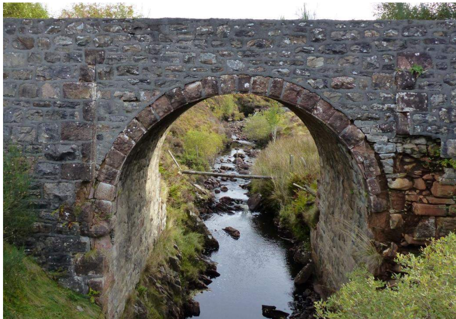
W face of the bridge (John Wombell)
