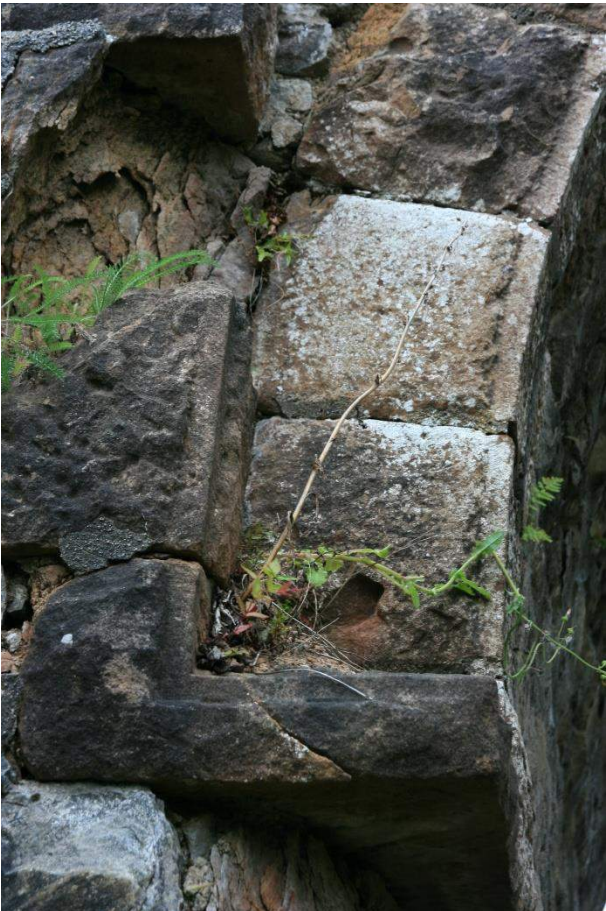
Detail of padstone, with rebated moulding, at base of NW spandrel (Janet Hooper)
