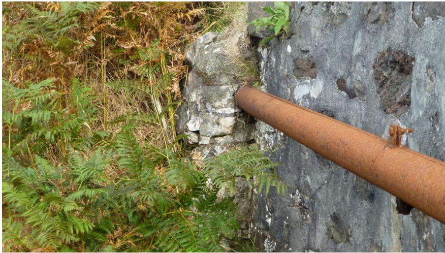
Buttress supporting pipe containing telephone cables on west side of bridge (Jock MacDonald)
