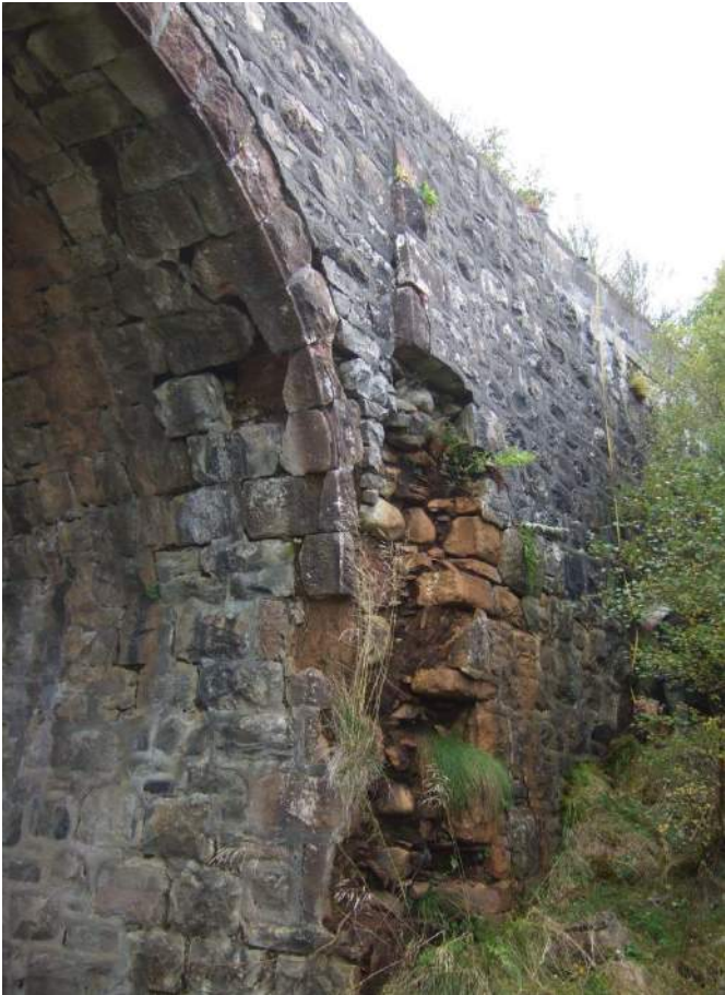
Damage to SW spandrel of bridge (Tom McCourt)
