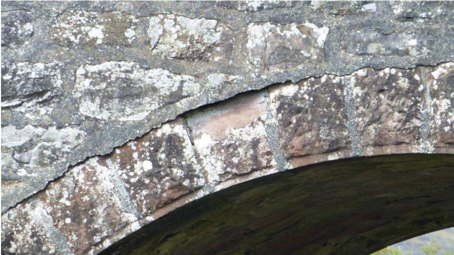
Detail of padstone, with rebated moulding, at base of NW spandrel (Janet Hooper)
