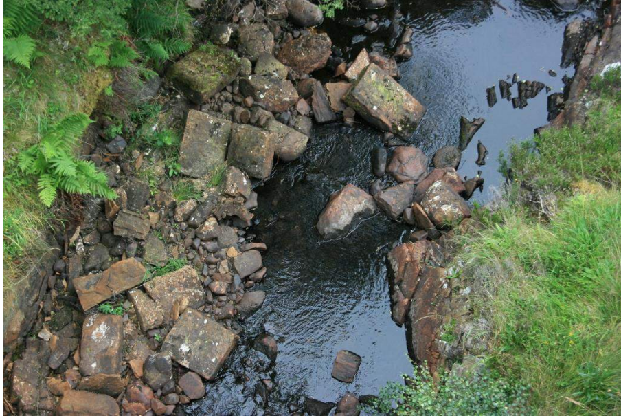
Dressed red sandstone blocks, which once formed the coping on the west side of the bridge, lying on the bed of the Allt na Fearn Mor (Janet Hooper)
