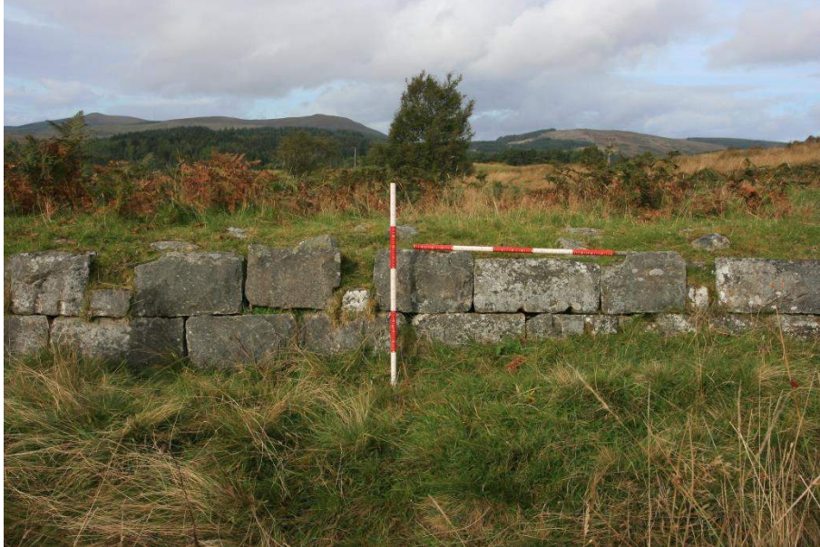
Dressed stone revetment on N bank of canalised burn (Janet Hooper)
